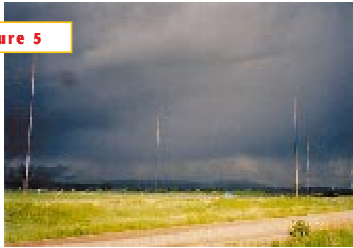
WWVB, which broadcasts at 60 kHz, requires multiple towers to support the large wire antenna.
