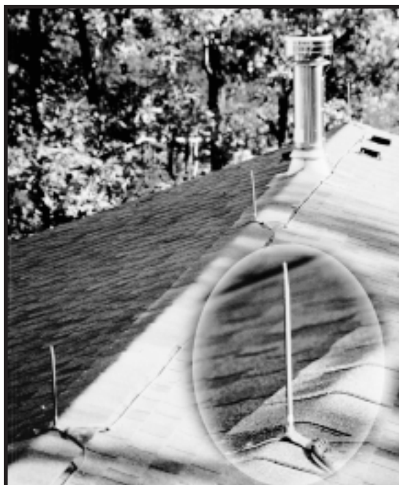
Photo 1 —Any effective lightning system starts with a good array of lightning rods spaced about every 20' along the peak. The insert shows one rod in a little closer detail.
