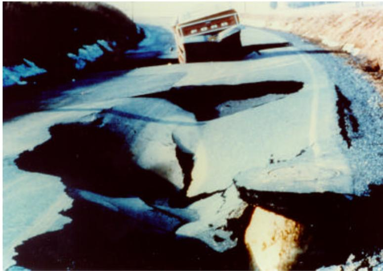
Figure 7- 1975 sinkhole related collapse under Bullfrog Valley Road, near Hershey, PA.
