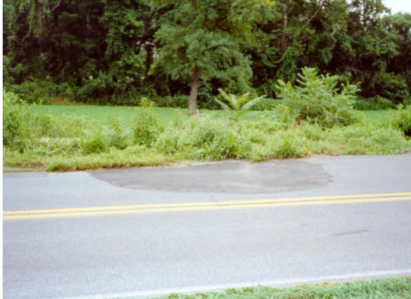
Figure 4 – Active sinkhole along Clifton Heights Road, Hummelstown, PA.
